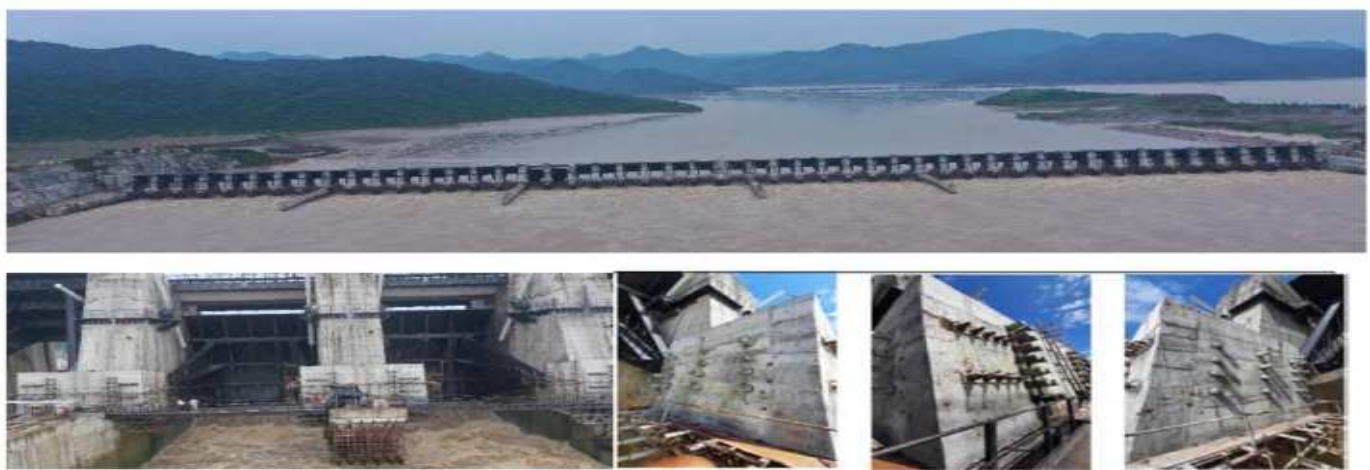
Fig.11. Integrity assessment of biaxially prestressed trunnion beams of dam structure
